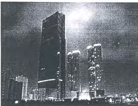
Keangnam Office Building Complex
